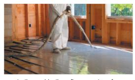
reduce noise and chafing, while providing a beautiful surface ready for your ceramic tile, marble tile or floor covering of your choice. The same sound and fire resistance qualities of our AccuCrete® underlayment products make AccuRadiant® the safe choice for your radiant heat installation.
