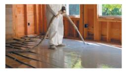
surface ready for your ceramic tile, marble tile or floor covering of your choice. The same sound and fire resistance qualities of our AccuCrete® underlayment products make AccuRadiant® the safe choice for your radiant heat installation.
