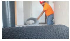
in multifamily construction where vinyl floor coverings allow applied loads to be passed directly through to the underlayment instead of being distributed over a larger area. Low deflection characteristics without sacrificing noise control, all in a low profile design.
